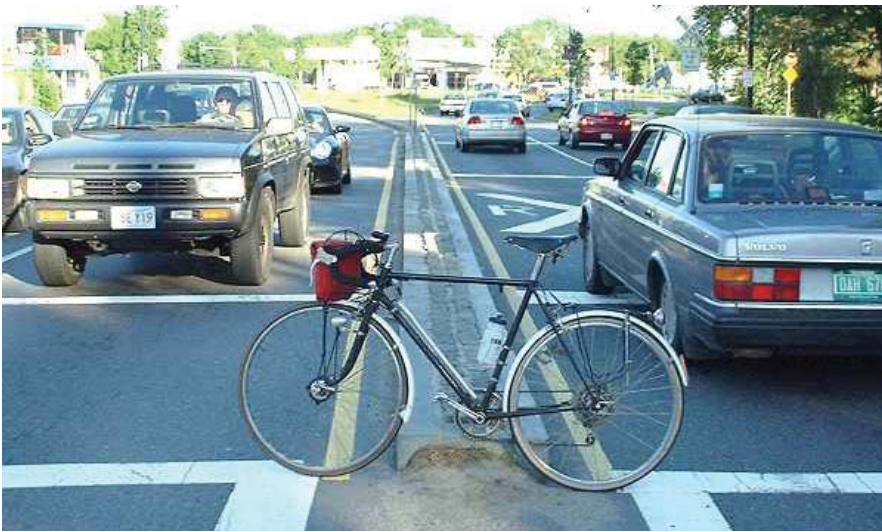
Figure 9.3: Medians must protect its users - wide enough for a bicycle, a stroller and a parent, a shopping cart, or a wheelchair
